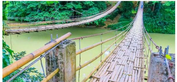
This 40 meter wide bridge was originally constructed by just using bamboo and rope, today the rope has been replaced by steel cables, giving added safety and stability
